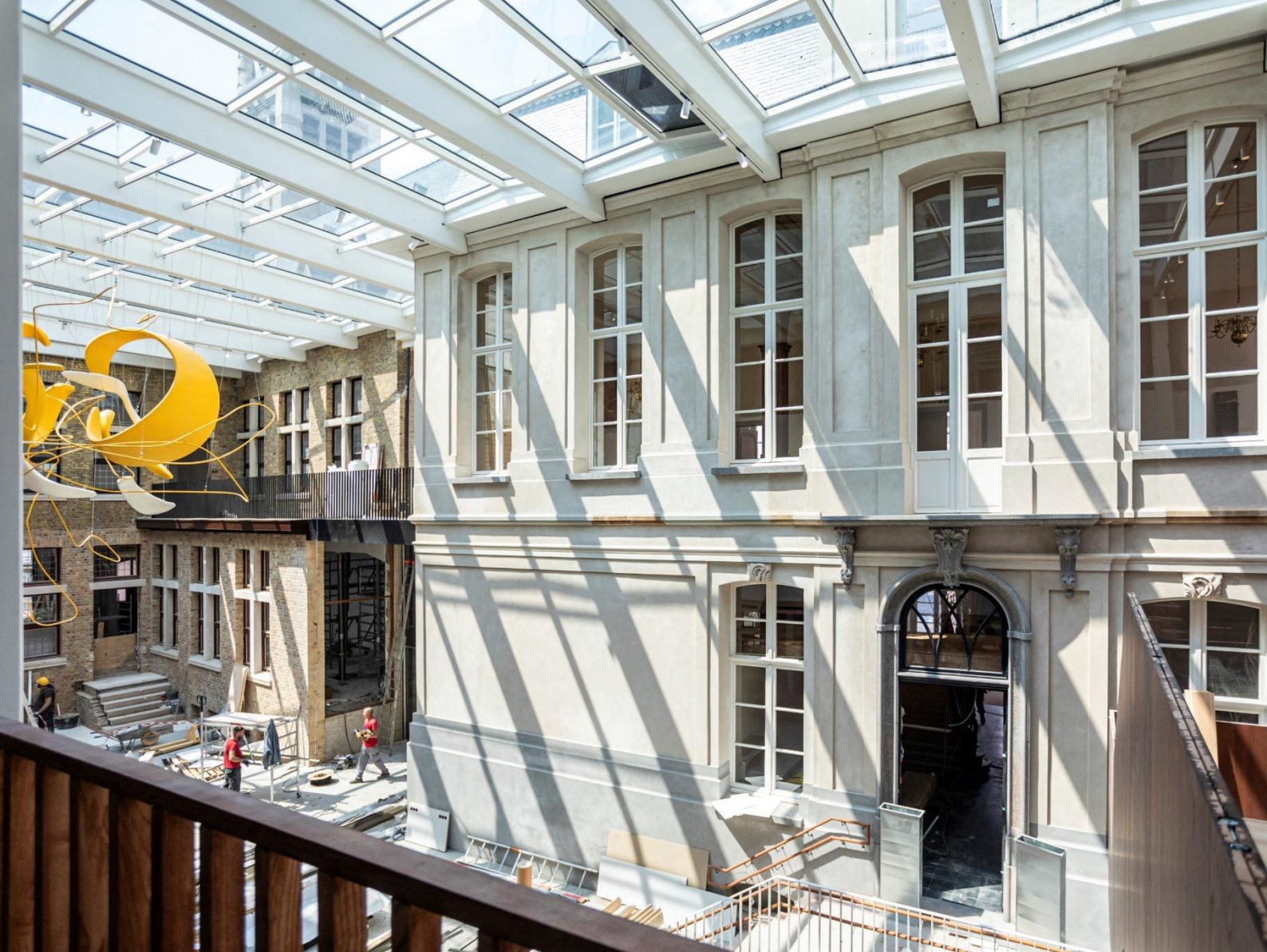
City hall Roeselare. © STUDIOPOINTU / Stad & OCMW Roeselare
